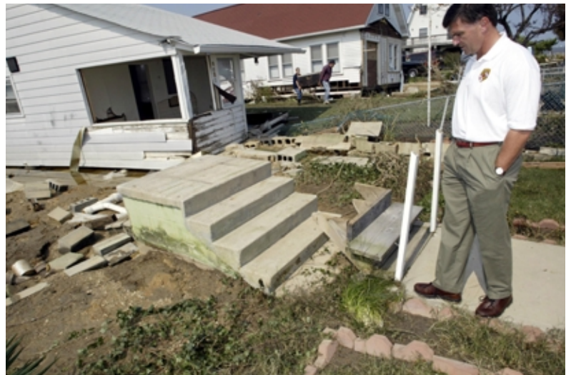
Maryland Governor Robert L. Ehrlich Jr. looks at a house knocked off of its frame by the winds of Hurricane Isabel on Atlantic Ave. while touring North Beach. The photo was taken by Post photographer MARK GAIL on Sept. 20.
