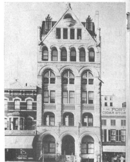
FIFTY YEARS AGO the present Post building was only a slight shadow of itself. Additions were made on sides and rear.
