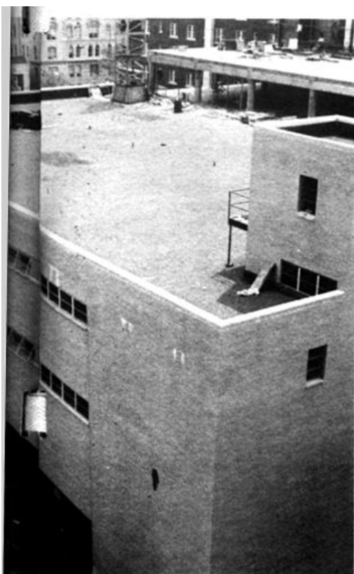
From the roof of the University Club on 16th Street, southwest corner of the building addition and the complex the rear of the Russian Embassy. The 5th floor is in the final state just behind the elevator penthouse.
