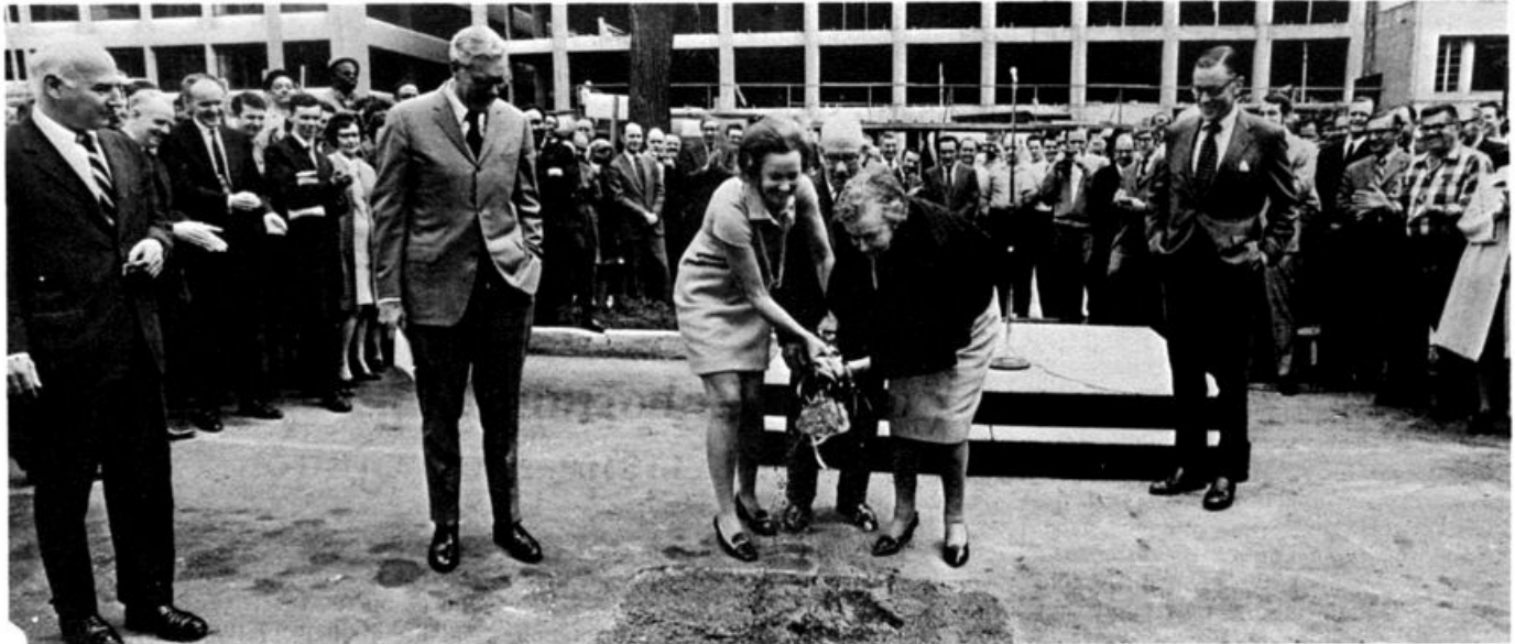
Mrs. Graham, Molly Parker and John Becker break ground for new Post building in ceremonies held April 17.
