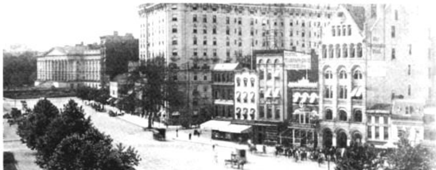
As shown in this 1905 photo, The Post building shared the neighborhood with several saloons, the Willard Hotel (large white building at left), and the Treasury Department (building with columns at far left).
