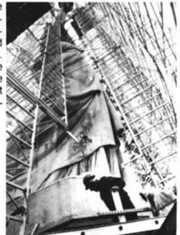
A worker is dwarfed by both the statue and the scaffolding.
